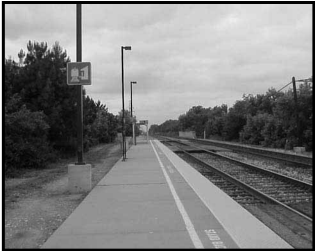
Amtrak Platform – Temporary Shelter
